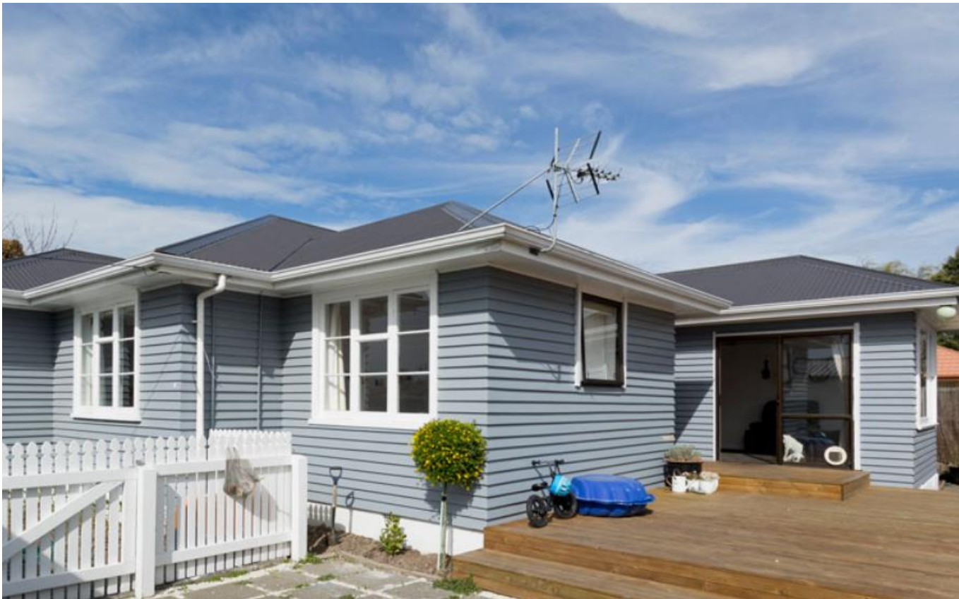
Ben & Quinn's renovation upgrade
